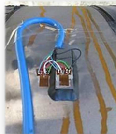
Tension measuring Installation of tensimeters
