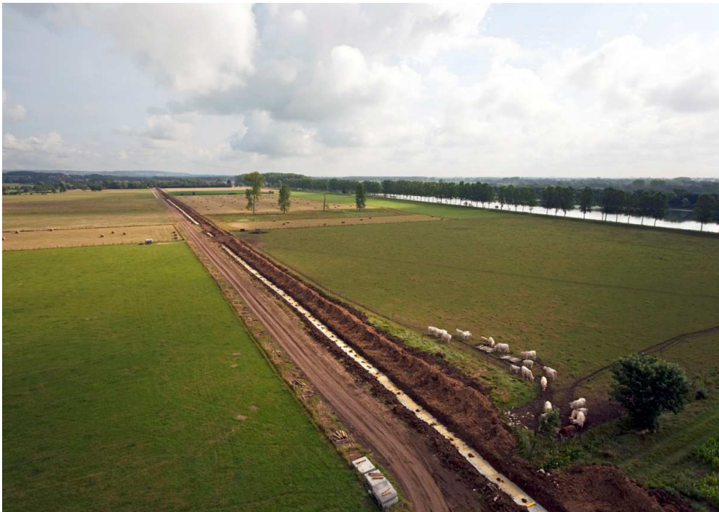
Figure 5.2 Sorting the types of soil excavated during trench digging
