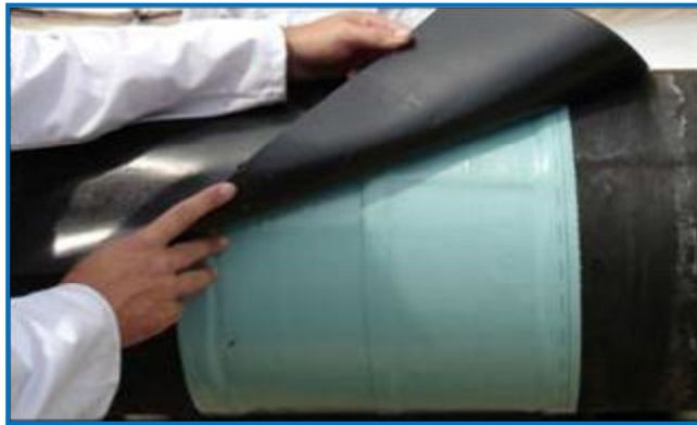
Figure 6.50 Polyisobutene tape with shrink cuff, installed on a transversal pipe weld
