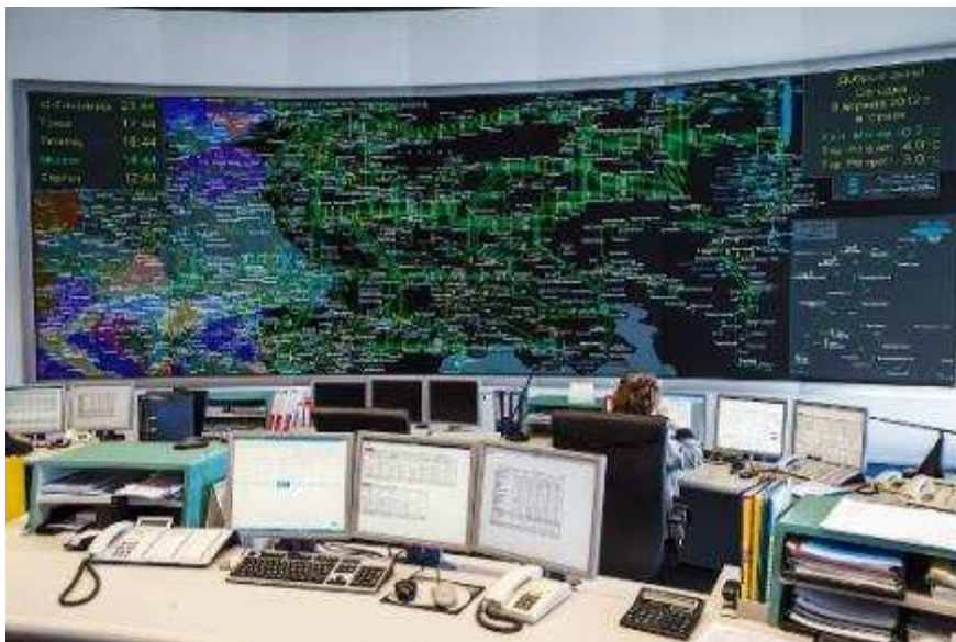
Figure 2.15 In Central Operations and Dispatch Department room (source: Gazprom)
