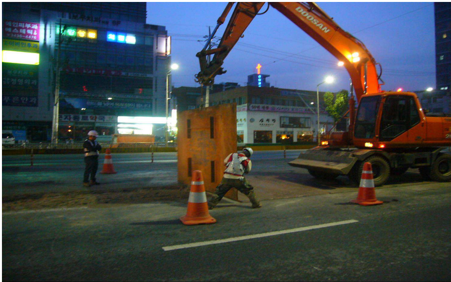
Figure 7.9 Works on the construction site
