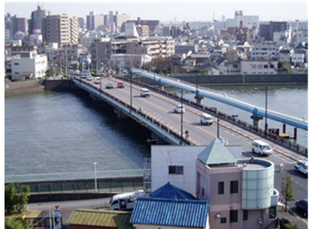
Figure 7.12 Typical scene along Chuo-Line route: crossing a river
